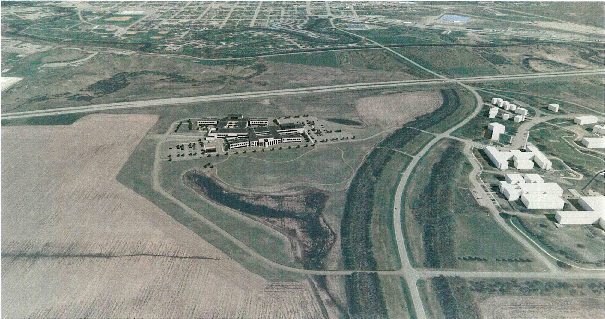
NORTH DAKOTA STATE HOSPITAL | OVERALL AERIAL VIEW FROM SOUTH
